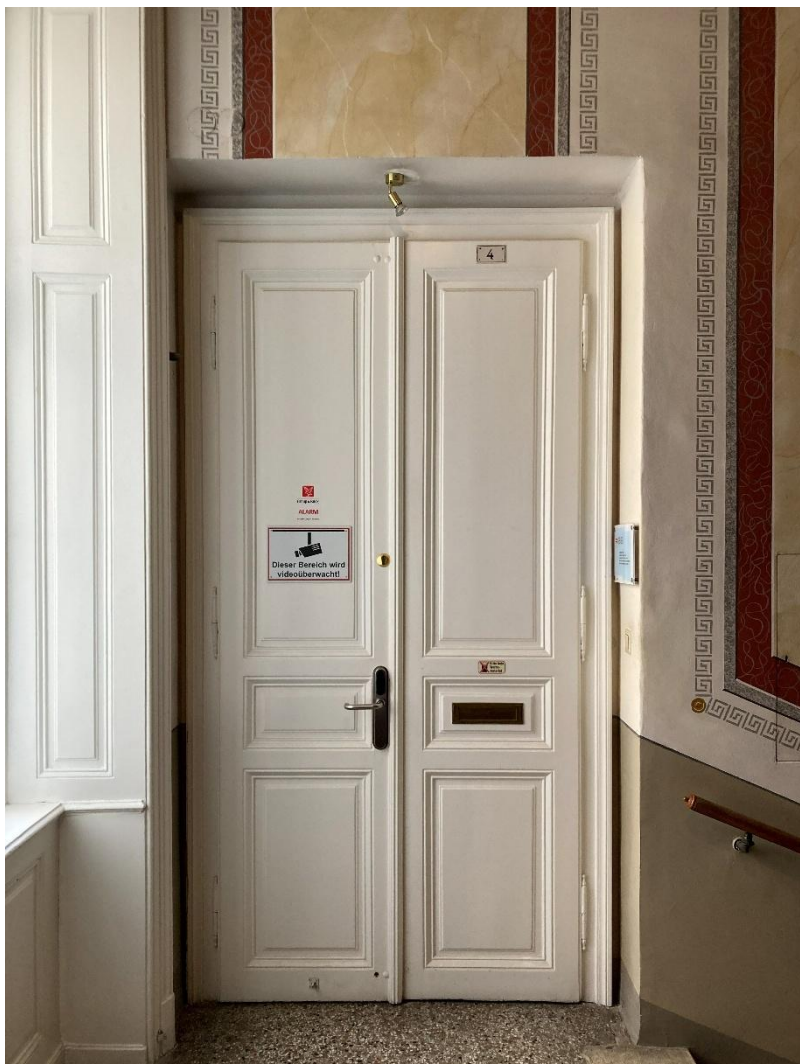
Figure5: Double doors on the mezzanine leading to reception
