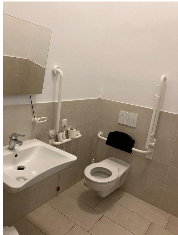
Figure 10: Interior view of the ladies' toilet on the mezzanine
