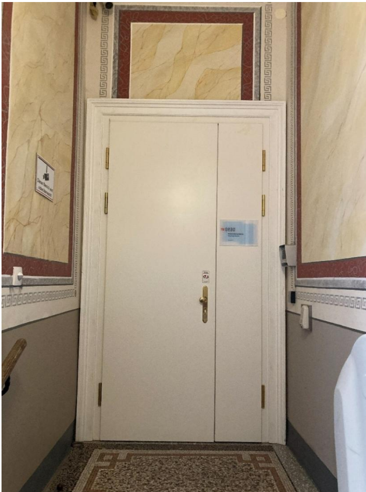
Figure7: Entrance door to the meeting room on the mezzanine
