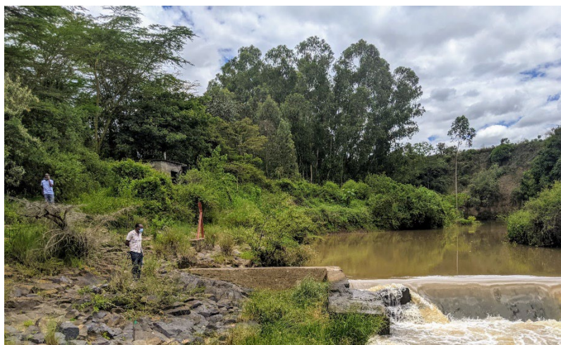
Figure 10: Malewa River gauging station (2GB05) (28.10.2021)
