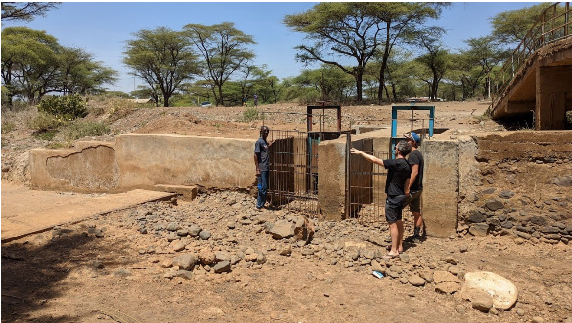
Figure 15: Waseges River gauging station 2EB10 in Sandai (top); Inlet for the Sandai irrigation scheme (bottom) (10.02.2022)
