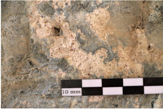
Fig. 7: Backfill mortar on ashlar masonry, cella, Water Temple
