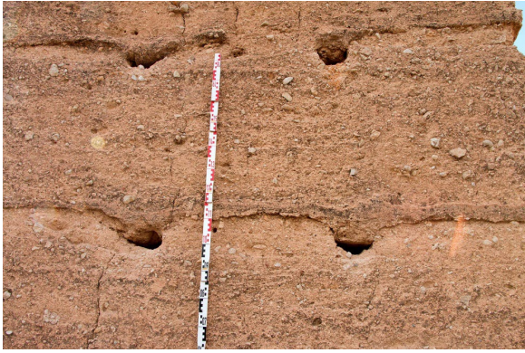
Fig. 37: Rammed-earth construction, Aqueduct
