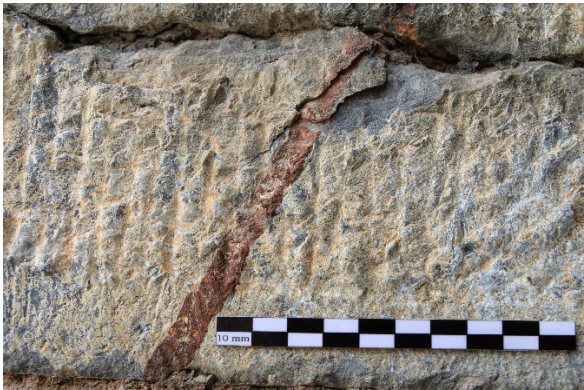
Fig. 3: Inclusions in gray limestone, red line, Water Temple
