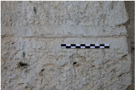
Fig. 17: White crust / deposit, ashlar masonry, wing, Water Temple Fig. 18: Black deposit / crust, cella wall exterior, Water Temple
