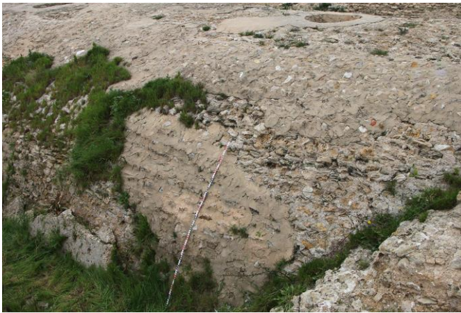
Fig. 32: restoration/reconstruction exterior, cisterns
