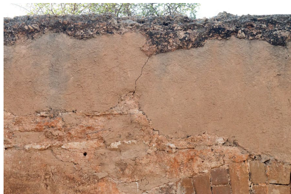
Fig. 47: Restoration intervention base zone of rammed-earth inventory, brown plaster and underneath restoration mortar, Aqueduct
