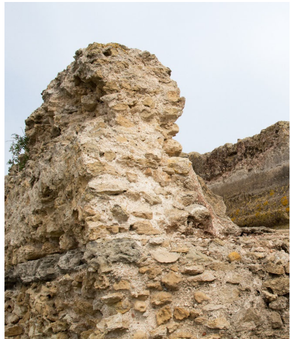
Fig. 5: aqueduct, row of grey stones below the sole of the specus
