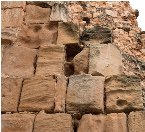
Fig. 53: Missing surface due to erosion of sand stone ashlar blocks, Aqueduct Fig. 54: Missing surface due to erosion of rammed-earth matrix, Aqueduct
