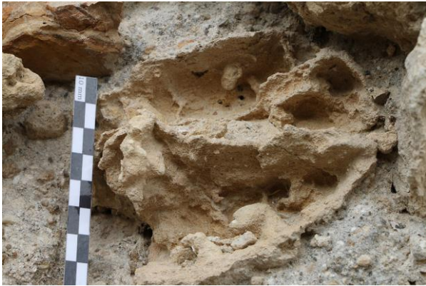
Fig. 34: sanding and alveolization masonry stone arch, cisterns
