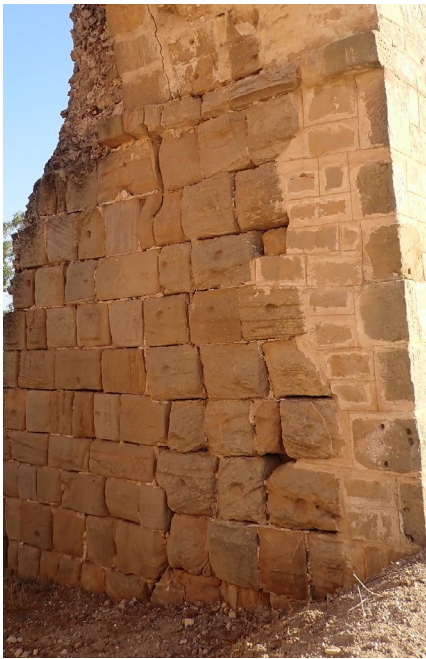
Fig. 33: Roman Ashlar masonry, middle part of wallstructure in this picture, Aqueduct
