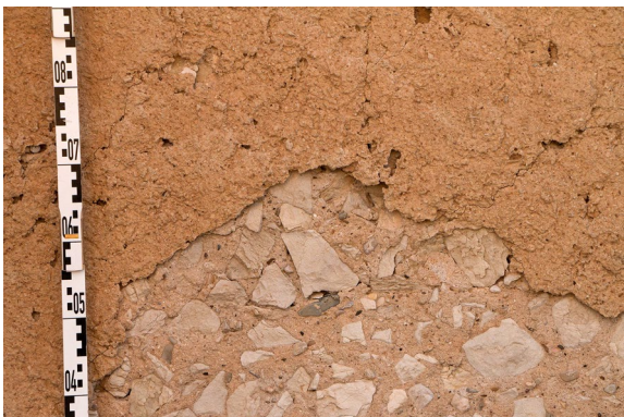
Fig. 47: Restoration intervention base zone of rammed-earth inventory, brown plaster and underneath restoration mortar, Aqueduct
