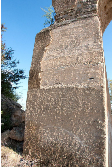
Fig. 49: Restoration intervention pillar no 12, reinforced concrete and brown plaster, Aqueduct Fig. 50: Crusts / Deposits on rammed-earth arch and pillar, Aqueduct
