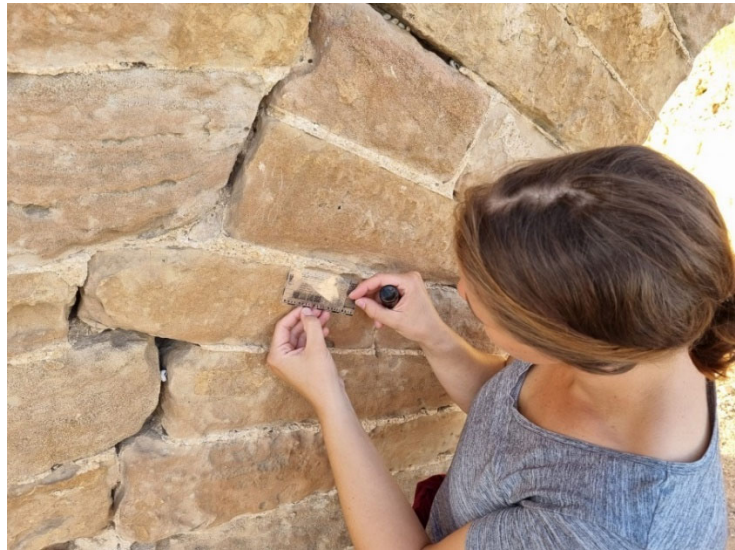
Fig. 2: Non-destructive material analyses on the aqueduct as part of the conservation-scientific inventory and condition survey (I. Mayer, ÖAW-ÖAI 2021)
