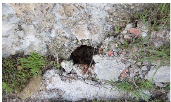
Fig. 7: cistern, drain channel between compartments 9 and 10 southern preserved section, on the vault of comp. 9; clay pipe is covered by opus signinum
