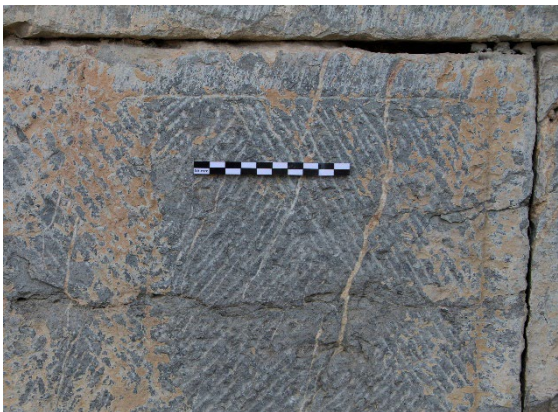
Fig. 5: Stonemasonry processing of gray limestone, fine geometrical lines, Water Temple
