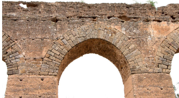
Fig. 39: Detail rammed-earth original surface preserved partially, Aqueduct
