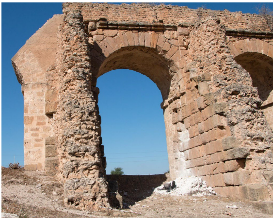
Fig. 41: Supporting walls, Aqueduct
