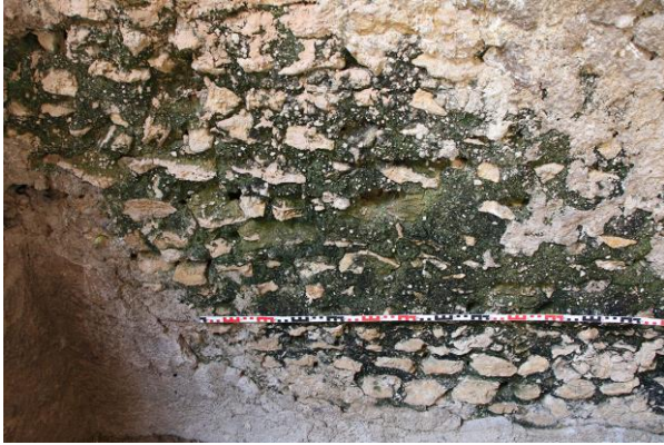
Fig. 36: biological colonization interior vault, cisterns
