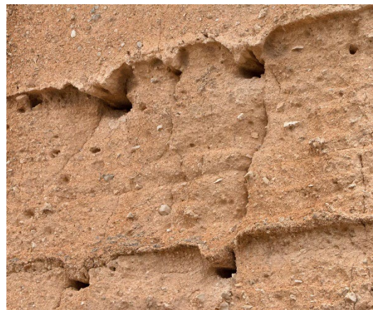
Fig. 53: Missing surface due to erosion of sand stone ashlar blocks, Aqueduct Fig. 54: Missing surface due to erosion of rammed-earth matrix, Aqueduct
