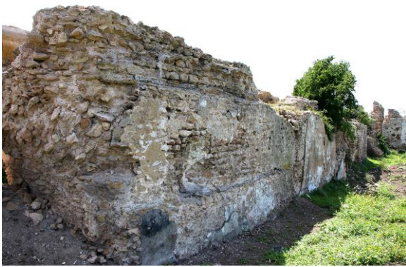
Fig. 9: re-use inventory, wall plaster on top of roman rubble stone wall
