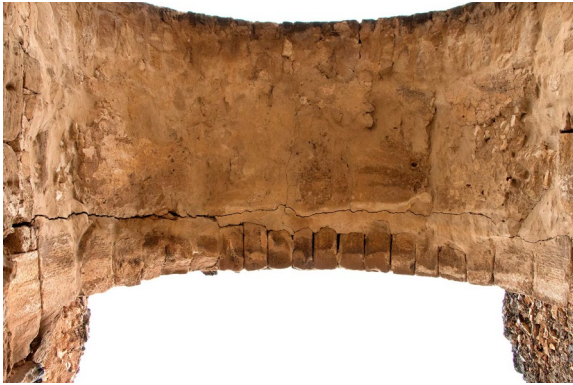
Fig. 51: Cracks between sandstone arch stones and rubble vault, Aqueduct Fig. 52: Biological Colonization arch and specus zone, plants as well as black biofilm and lichens, Aqueduct
