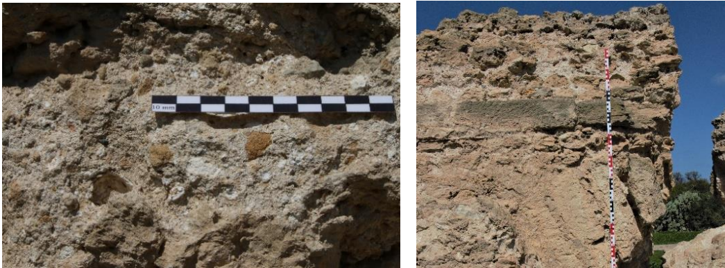
Fig. 3: roman inventory, mortar of opus caementitium wall structures
