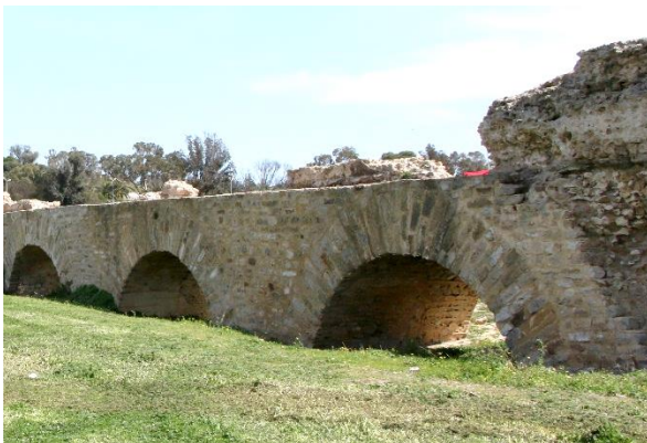
Fig. 11: restoration / reconstruction phase, reconstruction of vaults and spandrel walls north side
