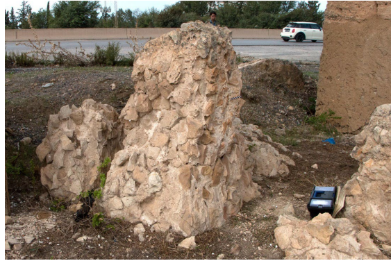
Fig. 44: Collapsed fragment of roman arch zone, opus caementicium core, Aqueduct
