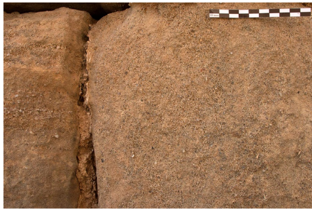
Fig. 33: Roman Ashlar masonry, middle part of wallstructure in this picture, Aqueduct
