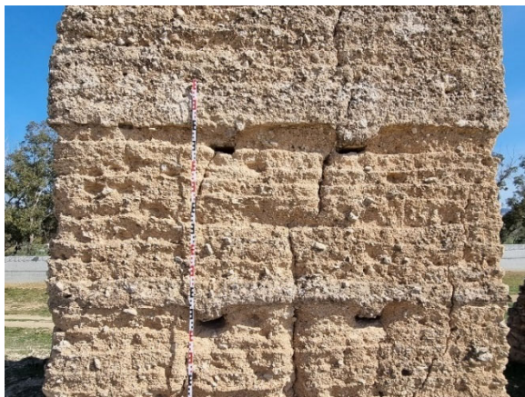
Fig. 6: Pillar 4 west face, rammed earth with levelling layers
