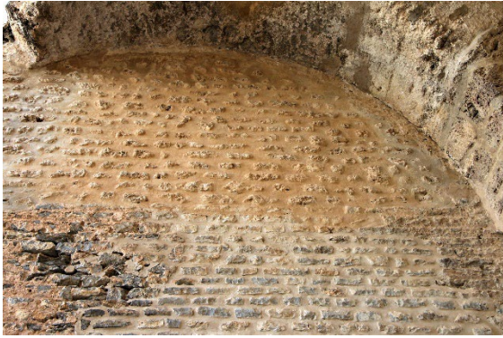
Fig. 15: Restoration interventions, restoration mortar, vault zone, Water Temple Fig. 16: Orange crust, ashlar masonry, wing, Water Temple
