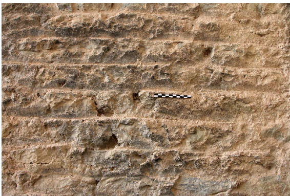
Fig. 13: Joint coating, cella wall, Water Temple
