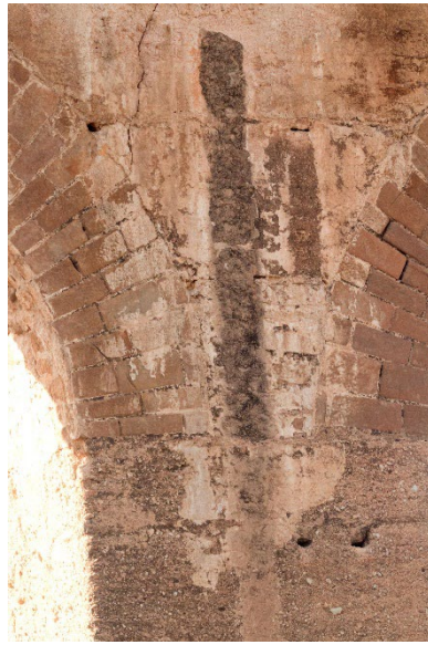
Fig. 49: Restoration intervention pillar no 12, reinforced concrete and brown plaster, Aqueduct Fig. 50: Crusts / Deposits on rammed-earth arch and pillar, Aqueduct
