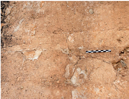
Fig. 39: Detail rammed-earth original surface preserved partially, Aqueduct
