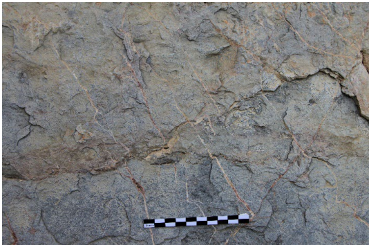
Fig. 19: Scaling, ashlar masonry, wing, Water Temple Fig. 20: Fragmentation, ashlar masonry, wing, Water Temple
