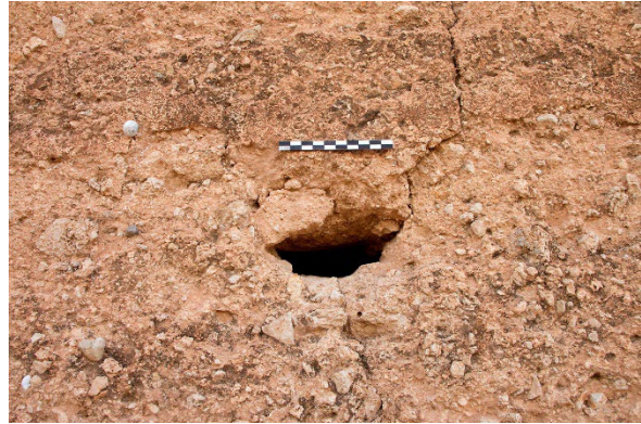
Fig. 38: Detail rammed-earth structure, putlog hole and interlayer (upperhalf of picture), Aqueduct
