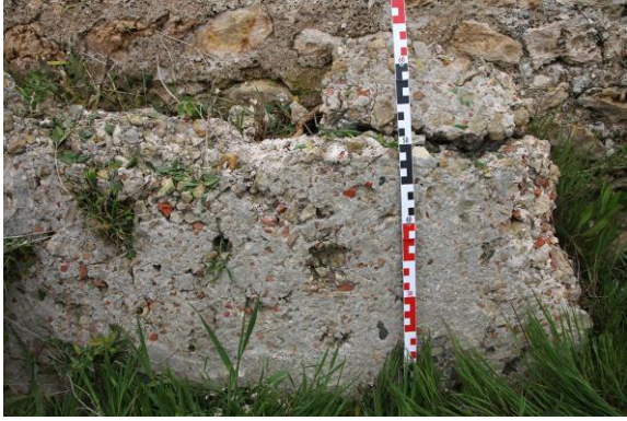
Fig. 30: plaster exterior drain channel, cisterns
