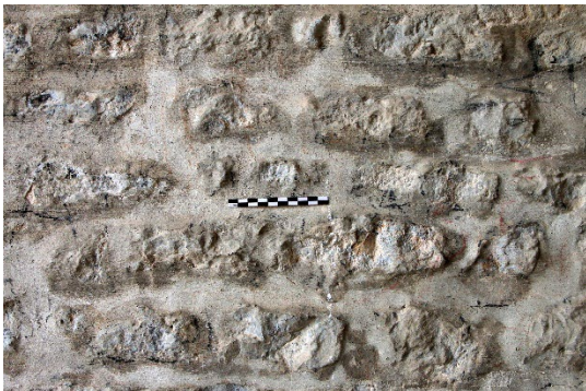
Fig. 25: Damp spots, possibly due to salts presence, rubble stone wall, cella interior, Water Temple
