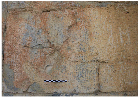
Fig. 15: Restoration interventions, restoration mortar, vault zone, Water Temple Fig. 16: Orange crust, ashlar masonry, wing, Water Temple
