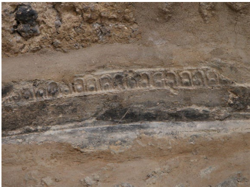
Fig. 11: Residues of decorative plaster, vault zone interior cella, Water Temple
