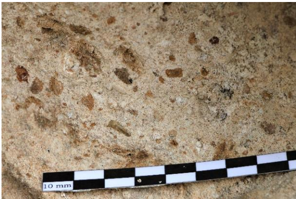
Fig. 28: mortar shield wall, cisterns
