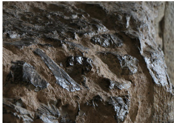
Fig. 25: Damp spots, possibly due to salts presence, rubble stone wall, cella interior, Water Temple
