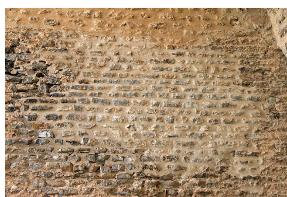
Fig. 14: Restoration interventions, new masonry, cella wall, Water Temple
