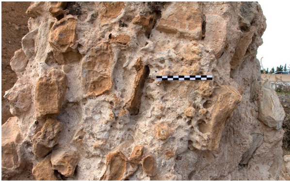
Fig. 45: Detail opus caementicium core, collapsed fragment, Aqueduct
