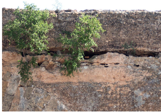
Fig. 51: Cracks between sandstone arch stones and rubble vault, Aqueduct Fig. 52: Biological Colonization arch and specus zone, plants as well as black biofilm and lichens, Aqueduct
