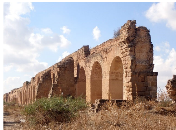
Fig. 2: A section of the Roman aqueduct structure in the Miliane Valley (G. Styhler-Aydın, OeAW-OeAI 2021)
