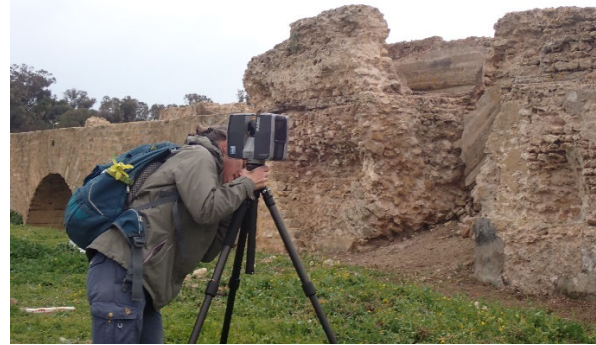
Fig. 10: Building survey of the aqueduct structure in Malga/Carthage (G. Styhler-Aydın, OeaW-OeAI Wien 2022)
