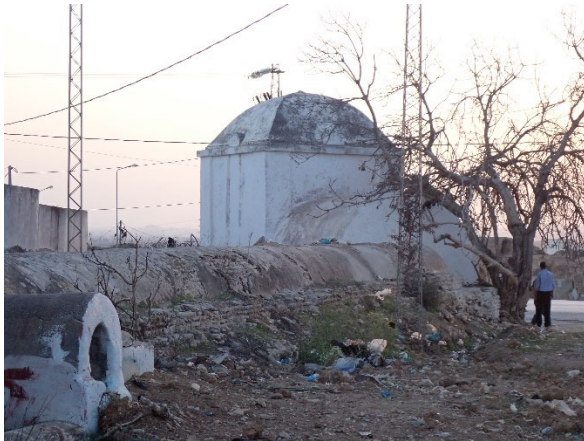
Fig. 3: The revitalized aqueduct structure of the 19 th century after the Miliane Valley (G. Styhler-Aydın, OeAW-OeAI 2021)
