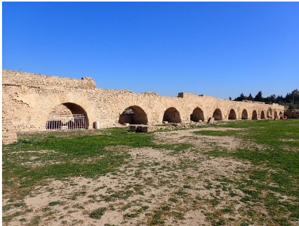
Fig. 5: A section of the aqueduct structure in the area of the Malga cistern in Carthage (G. Styhler-Aydın, OeAW-OeAI
