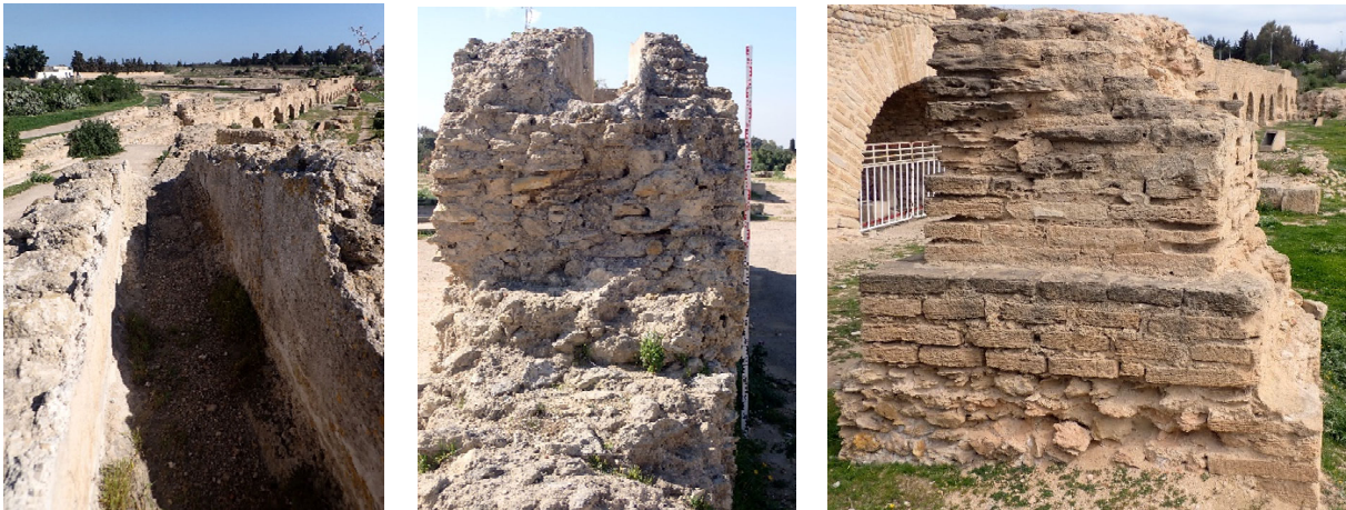
Fig. 13a-c: Area of Malga/Carthage. Secondary built aqueduct structures (left, middle). Reused material from the ancient aqueduct for pipeline pillars of a later construction phase (G. Styhler-Aydin, OeaW-OeAI Wien 2022)
