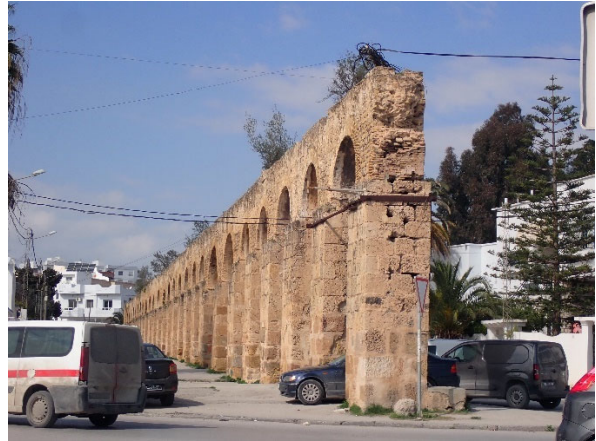
Fig. 4: A section of the aqueduct structure at the level of the Bardo in today's Tunis (G. Styhler-Aydın, OeAW-OeAI 2022)
